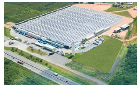
The new Marcegaglia plant in Garuva (Santa Catarina)
